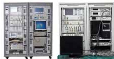
ATE ATS FACILITY
