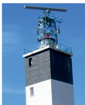
Coastal Surveillance System
